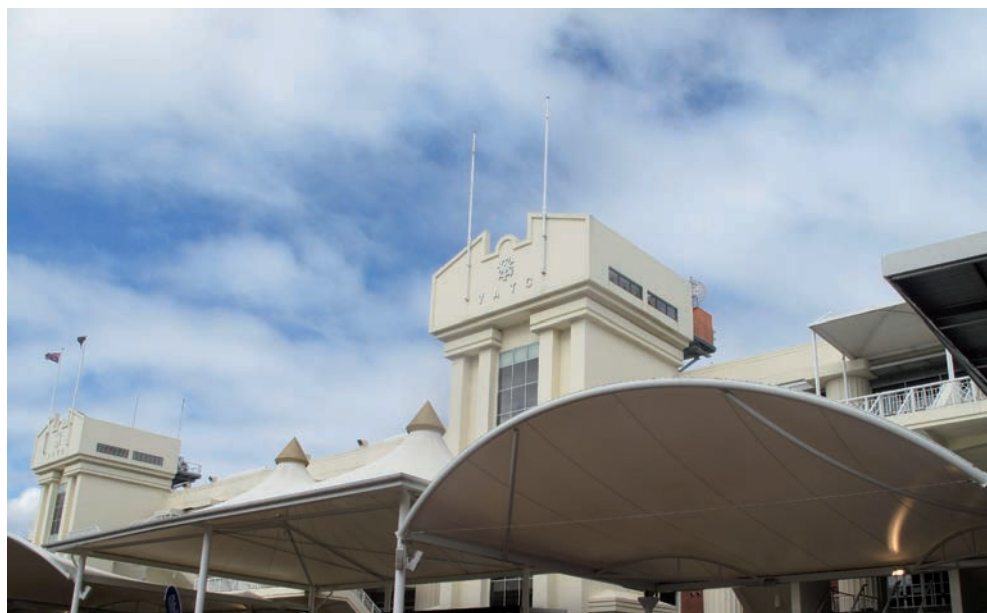
Caulfield Racecourse concourse (Image: Eric Frazer)
