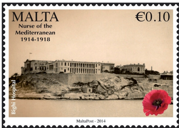
Figure 3: Bighi Hospital had quite large corridors ideal for shielding patients from the summer midday sun and inclement weather while the wards had high ceilings. Due to the huge numbers of patients, at one point, they were bedded in corridors and ditches.
