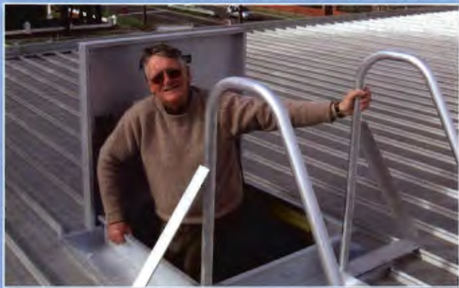
President John Shawley inspects the newly-installed roof ladder to Purves House.
